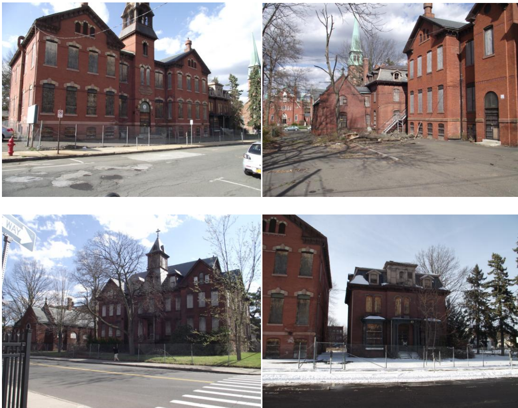
Figure 16 - Existing Conditions of Catholic School Buildings
