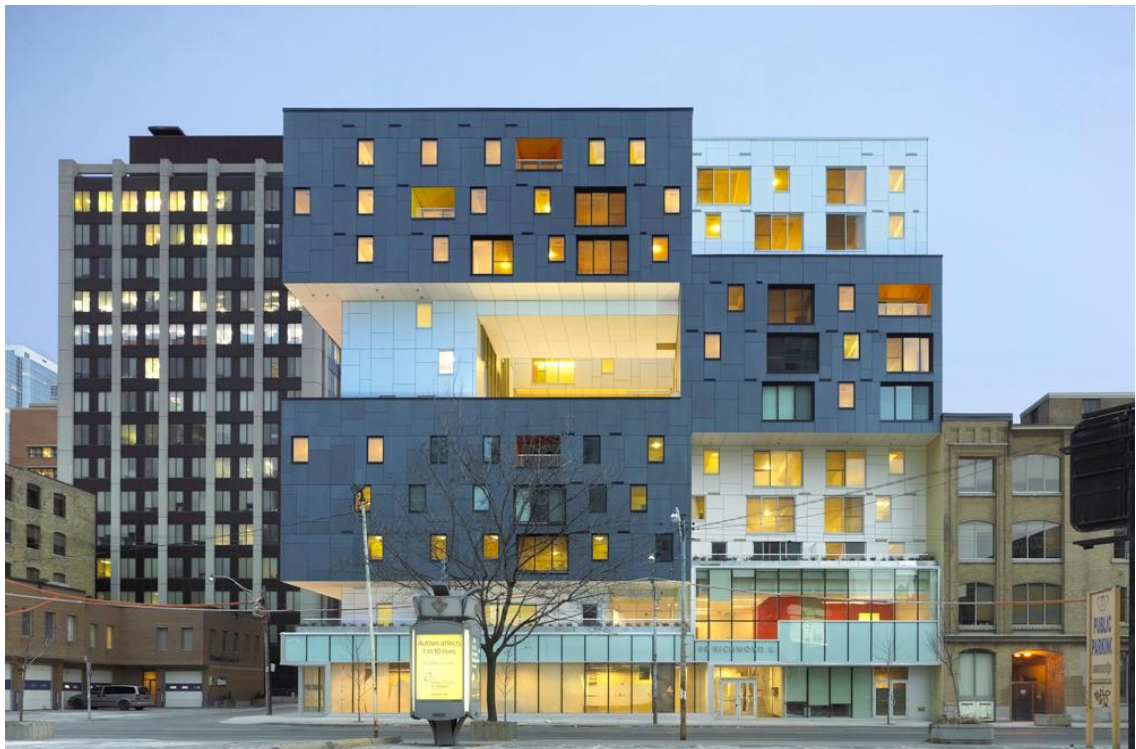
Figure 5 - Photograph of Primary Facade at 60 Richmond
