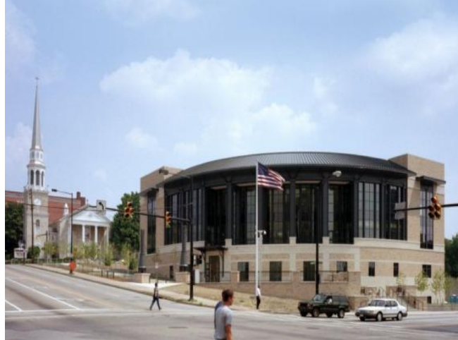
Figure 1 - Nathaniel R. Jones Federal Building
