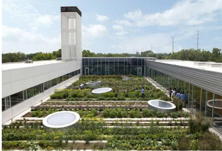
Figure 9 - Aerial Photograph of Roof Garden
