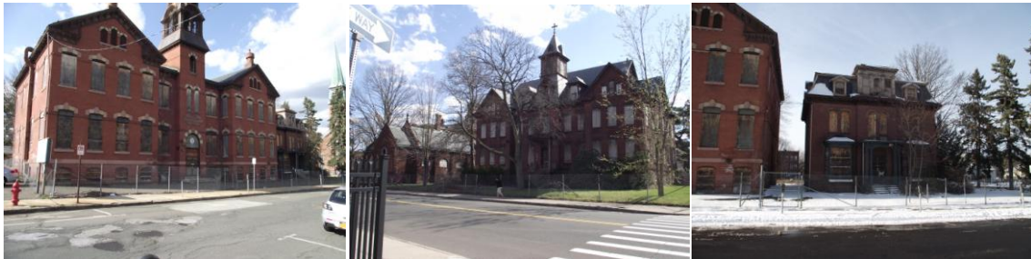
Figure 30 - Existing Catholic School Buildings on Site
